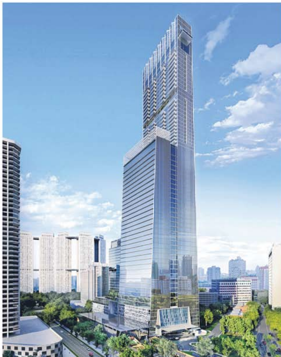
Artist's impression of the Tanjong Pagar Centre. The project is on schedule to receive Temporary Occupation Permit in July 2016.
