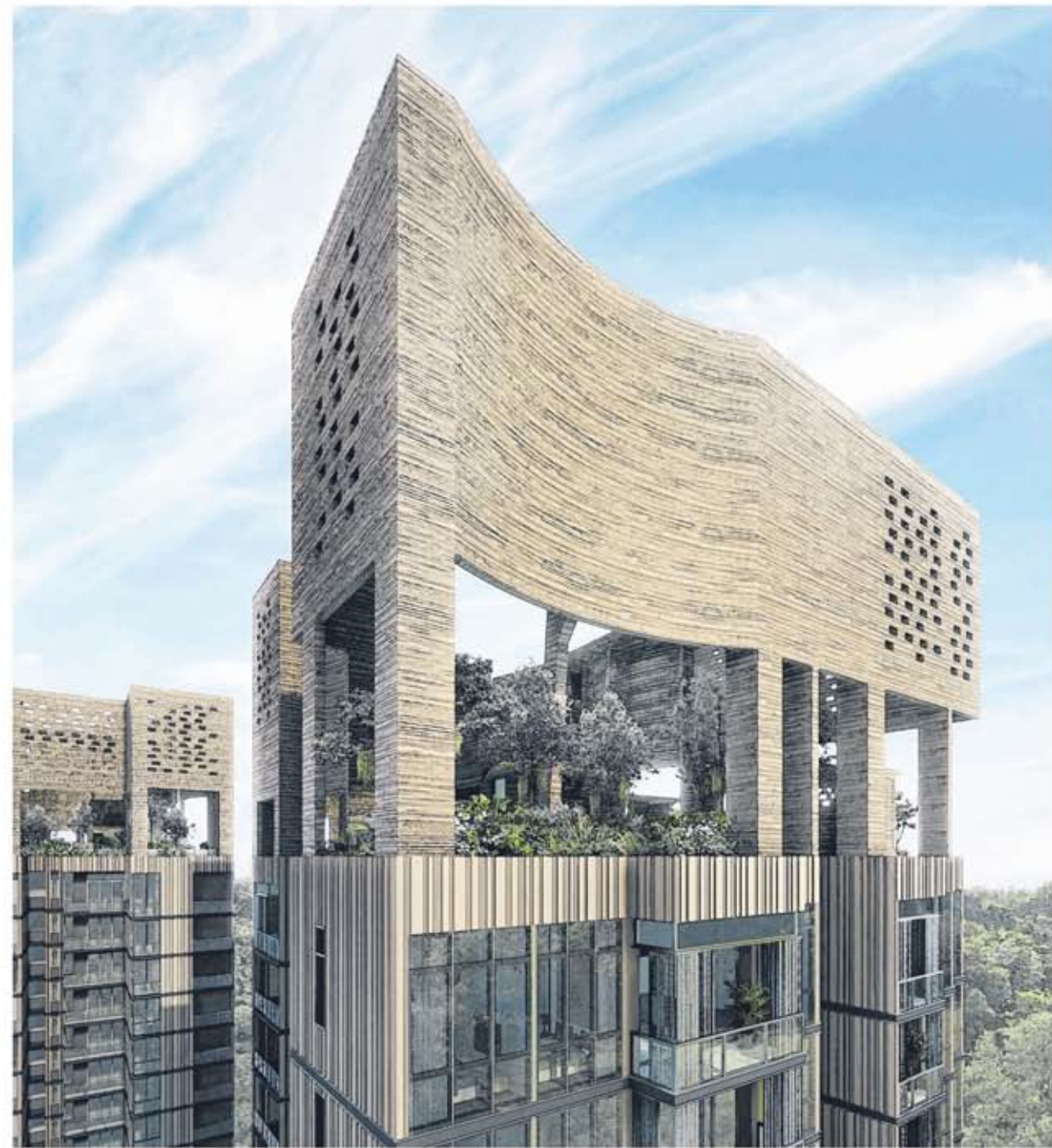
Martin Modern's two 30-storey towers will house 450 apartments and should be completed by 2022. Half the buyers are expected to be owner-occupiers, and the other half, investors. PHOTO: COURTESY OF GUOCOLAND GROUP
