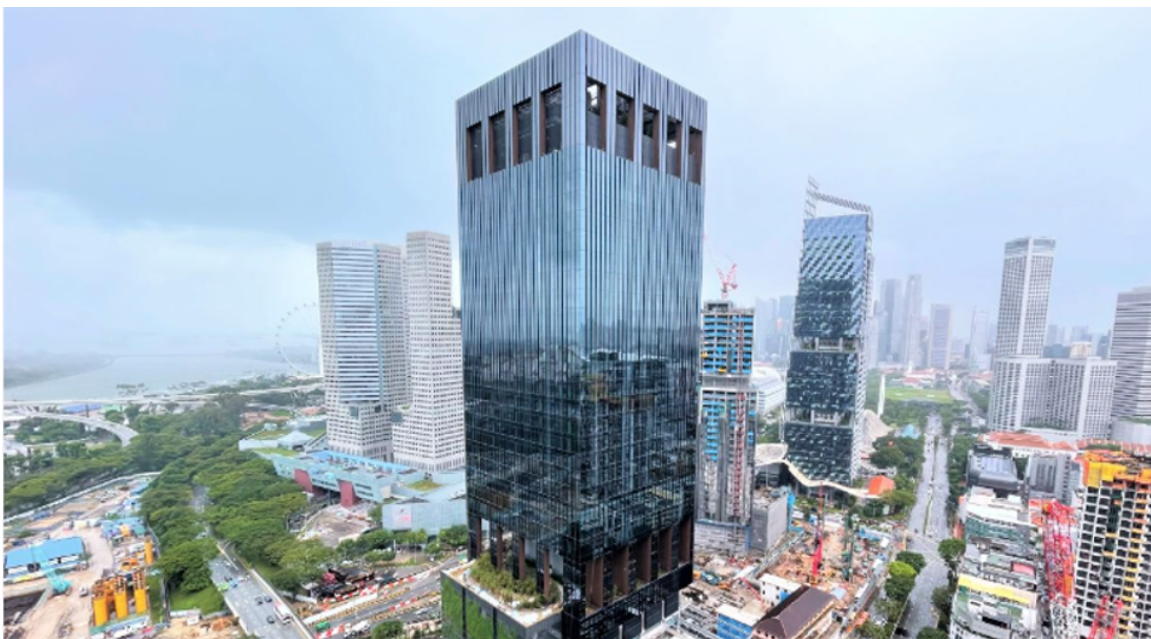
Guoco Midtown's office tower GuocoLand
