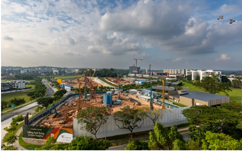
The construction taking place at Lentor Hills estate, created from a greenfield site
